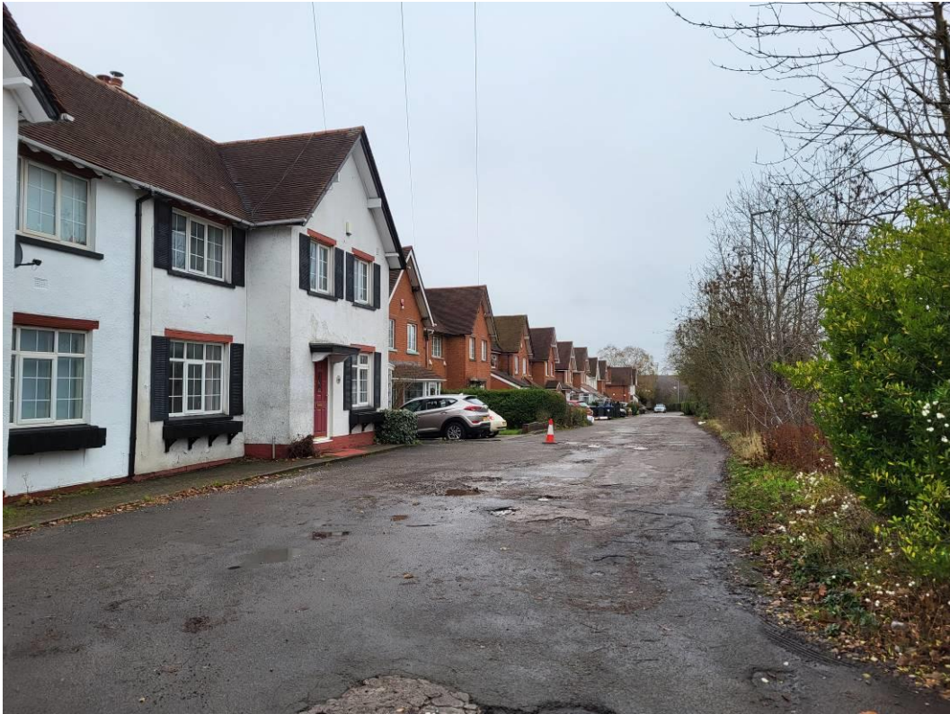
Plate 7: Looking east along The Crescent service road
