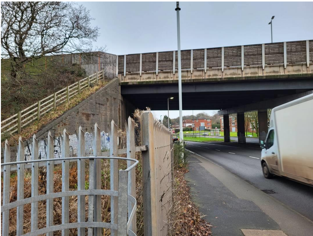
Plate 12: The M6 bridge over Queslett Road immediately east of the entrance to the footpath
